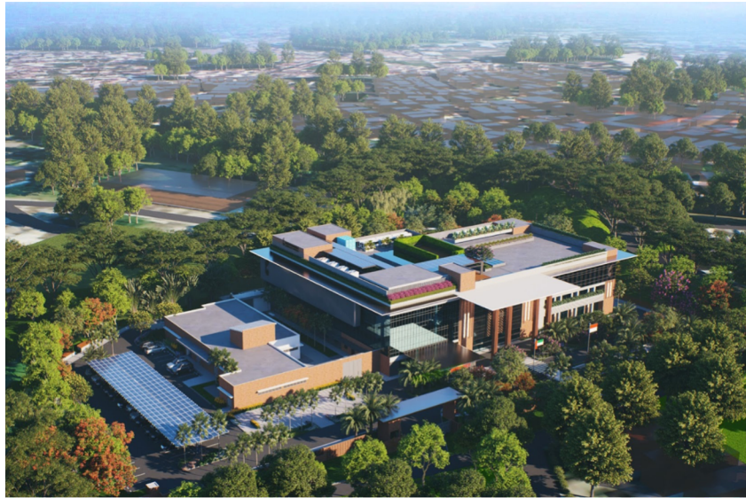
The Emirates-Indonesia Cardiology Hospital in Solo Technopark by Government of UAE
